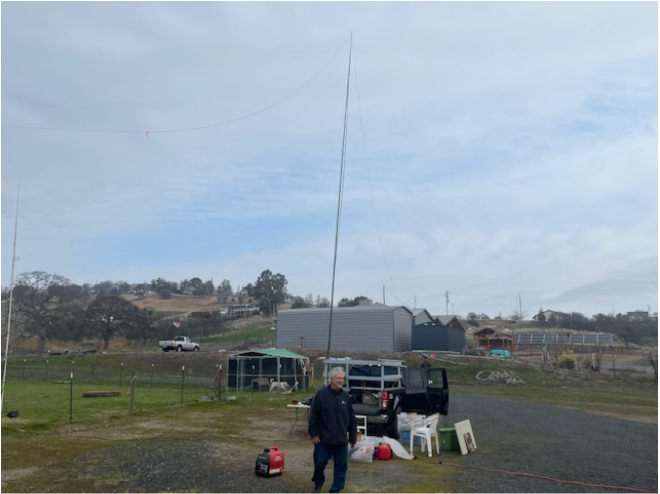
K06F0V surveying the site
